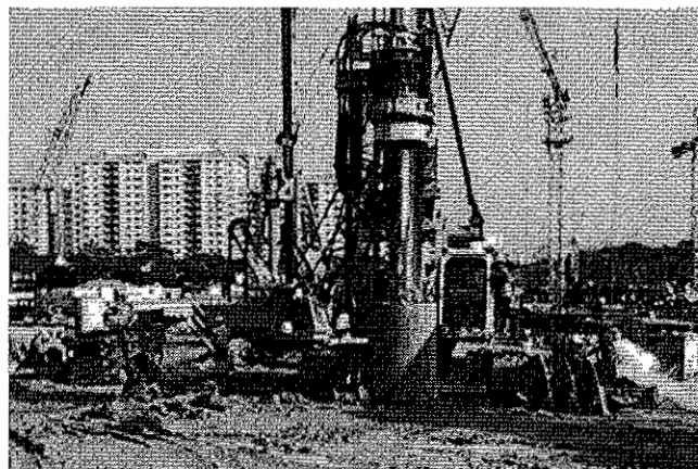
Piling works for Paradigm Mall, a mixed development located at Kelana Jaya, Selangor as undertaken by our Group
