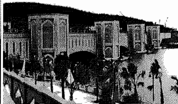
Arch beam bridge in Putrajaya as constructed by our Group
